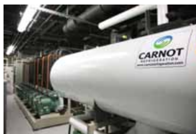
Fig. 2 Photos of the transcritical CO 2 system at Sobeys designed by Carnot Refrigeration.
